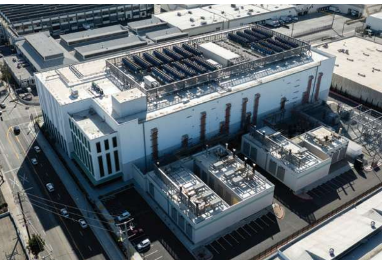
◀ Data center facility, Vernon, California.
